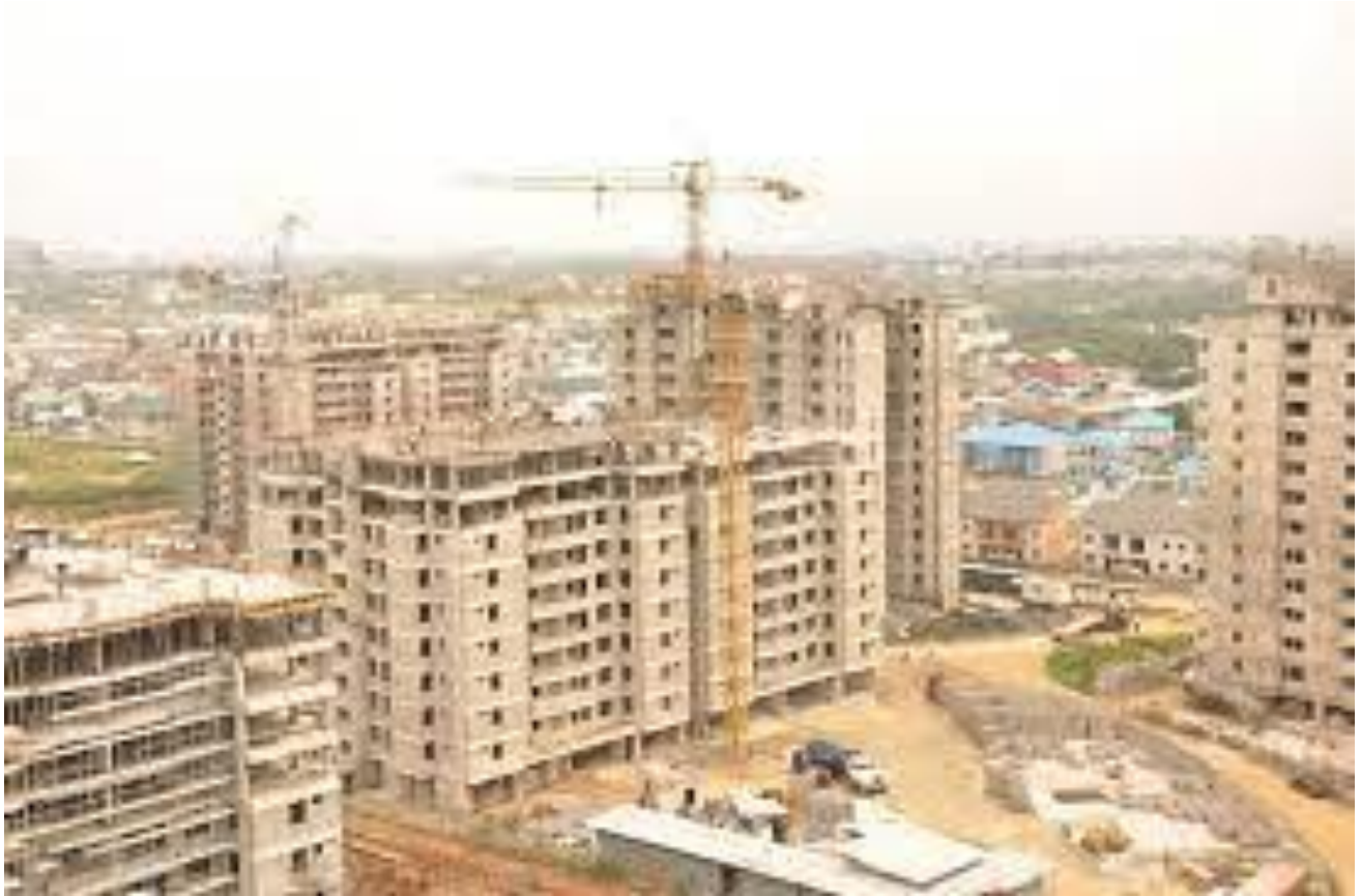
Figure 3: Picture showing construction work of housing development in Rainbow Town
